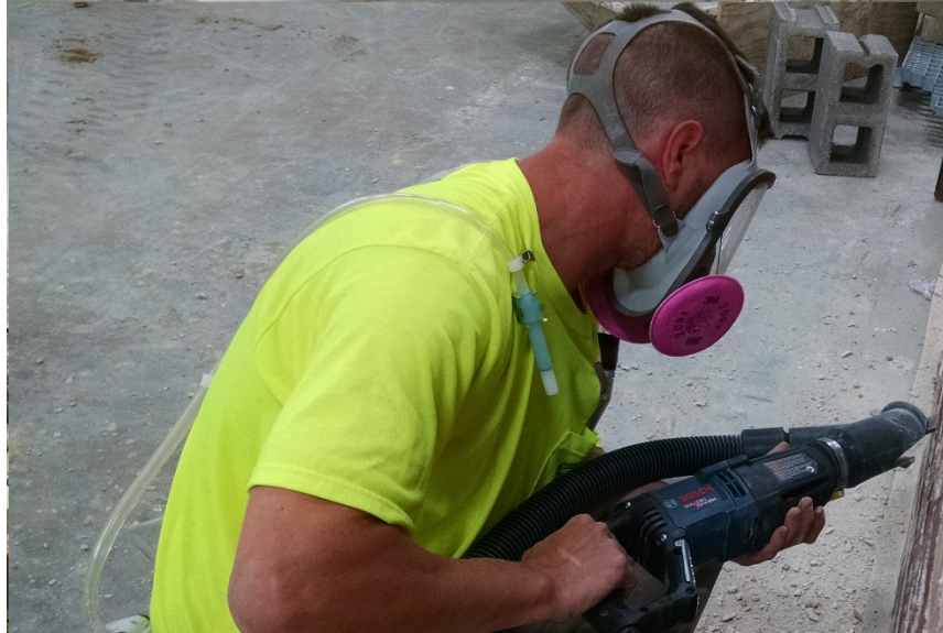
Figure 6 – SidePak cyclone in the worker’s breathing zone (NIOSH photo)
