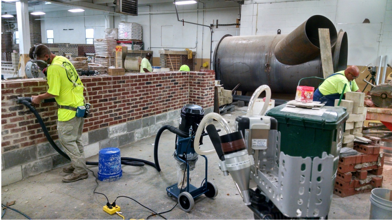
Figure 7 – Instructor Sawing Brick. The Area Sampler is Visible Behind Him (NIOSH photo).
