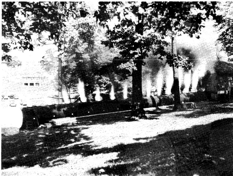
FIGURE 7. - Former gallery for testing explosives at Bruceton, PA. Here, black powder—a nonpermissible explosive—produces a violent explosion.
