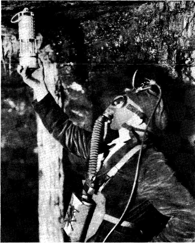
FIGURE 5. - Early test for methane gas in the Experimental Mine using flame safety lamp.
