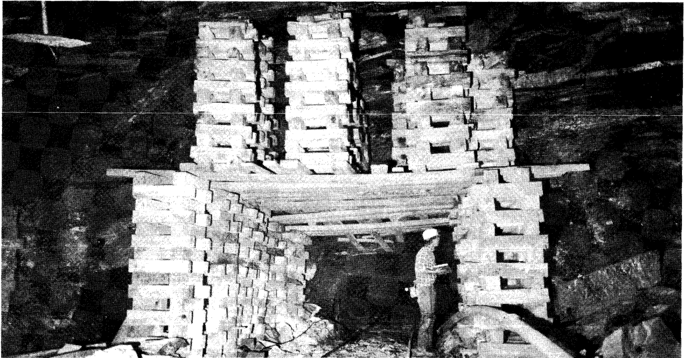
FIGURE 9. - Conducting a geologic study in a coal mine roof fall area.
