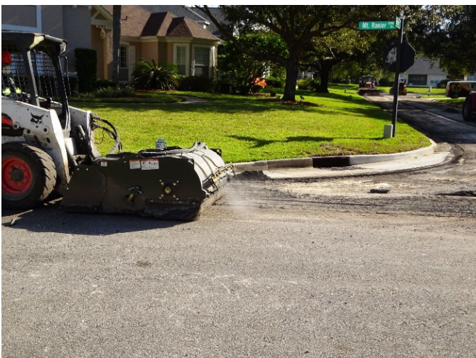
Figure A13. Water-based dust suppression attachment being used to sweep freshly-milled road surface prior to re-paving. No substantial dust generation was observed. Photo by NIOSH.
