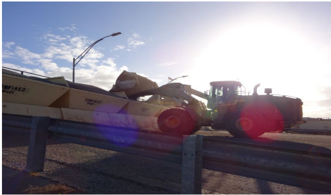
Figure A5. Front end loader with enclosed cab used to load raw materials into hoppers that feed the asphalt production plant via the conveyor belt system. Photo by NIOSH.
