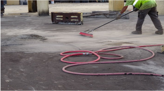
Figure A2. Worker dry sweeping yard beneath asphalt production plant. Photo by NIOSH.
