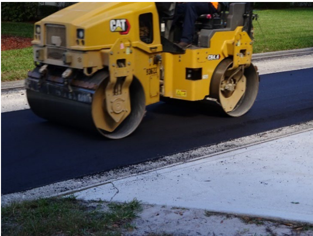
Figure A15. Asphalt roller used to smooth surface. Photo by NIOSH.
