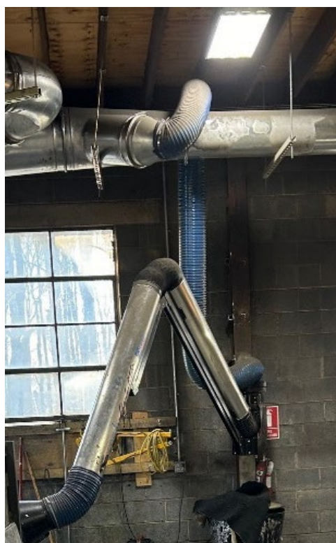
Figure B3. Movable flexible "elephant trunk" style LEV hood attached via corrugated plastic ductwork to the permanent hard metal duct. Photo by NIOSH.
