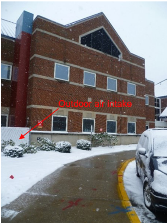
Figure A2. View of potential pollutant sources for outdoor air intake. Photo by NIOSH.
