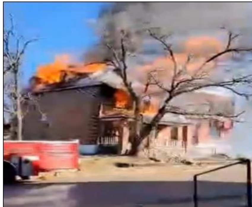
Conditions on the arrival of Truck 13 showing post flashover fire conditions throughout the second and third floors. Photo courtesy of FD.
