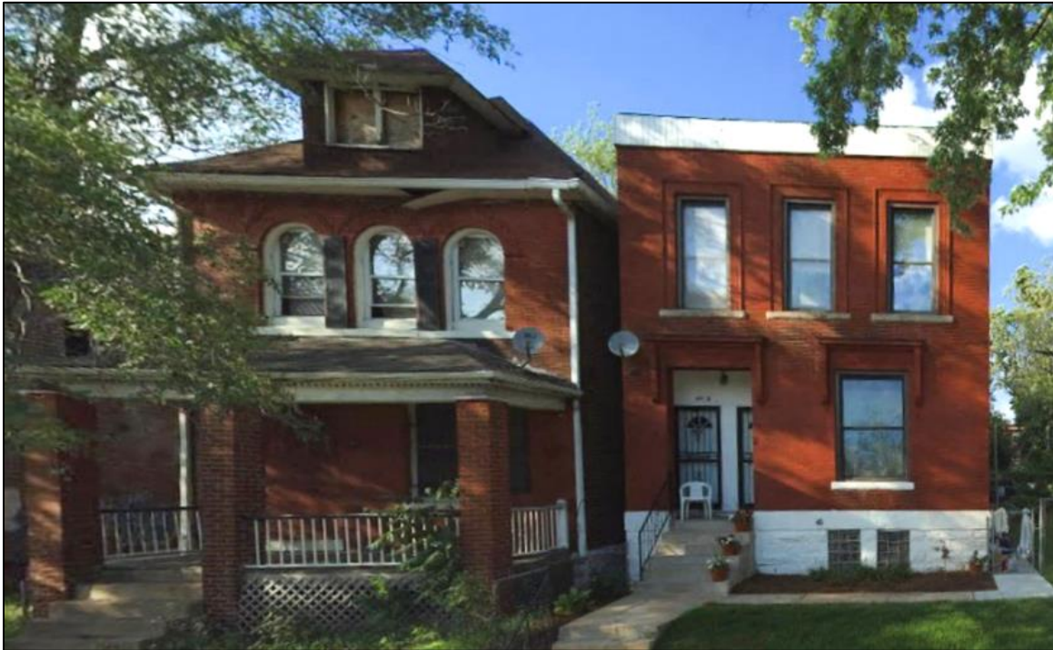
Photo 2. Fire building on the left, and the Side Delta exposure on the right, showing pre-fire conditions. Note indications of the fire building being a derelict structure with deteriorated conditions. (Photo from Google Earth)
