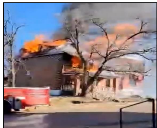
Photo 1. Conditions on the arrival of Truck 13 showing post flashover fire conditions throughout the second and third floors. (Courtesy of FD)
