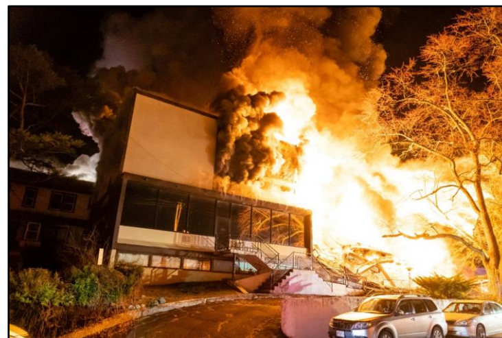
The cantilever collapse of Side Bravo/Side Charlie corner of the original building. The time was approximately 02:08 hours. (Photo Courtesy of Kenneth Flynn)
