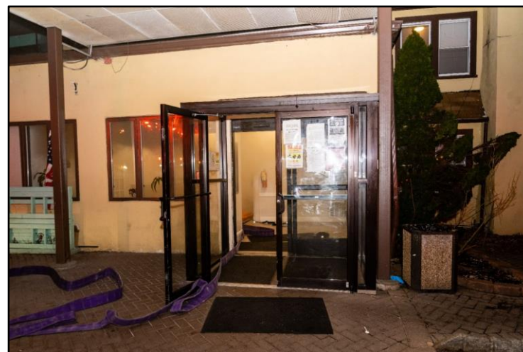
Photograph of smoke condition observed in the lobby. The 3-inch hoseline from Tanker 17 was stretched up the stairwell to the 2 nd floor. The time was approximately 01:12 hours. (Photograph courtesy of Kenneth Flynn)
