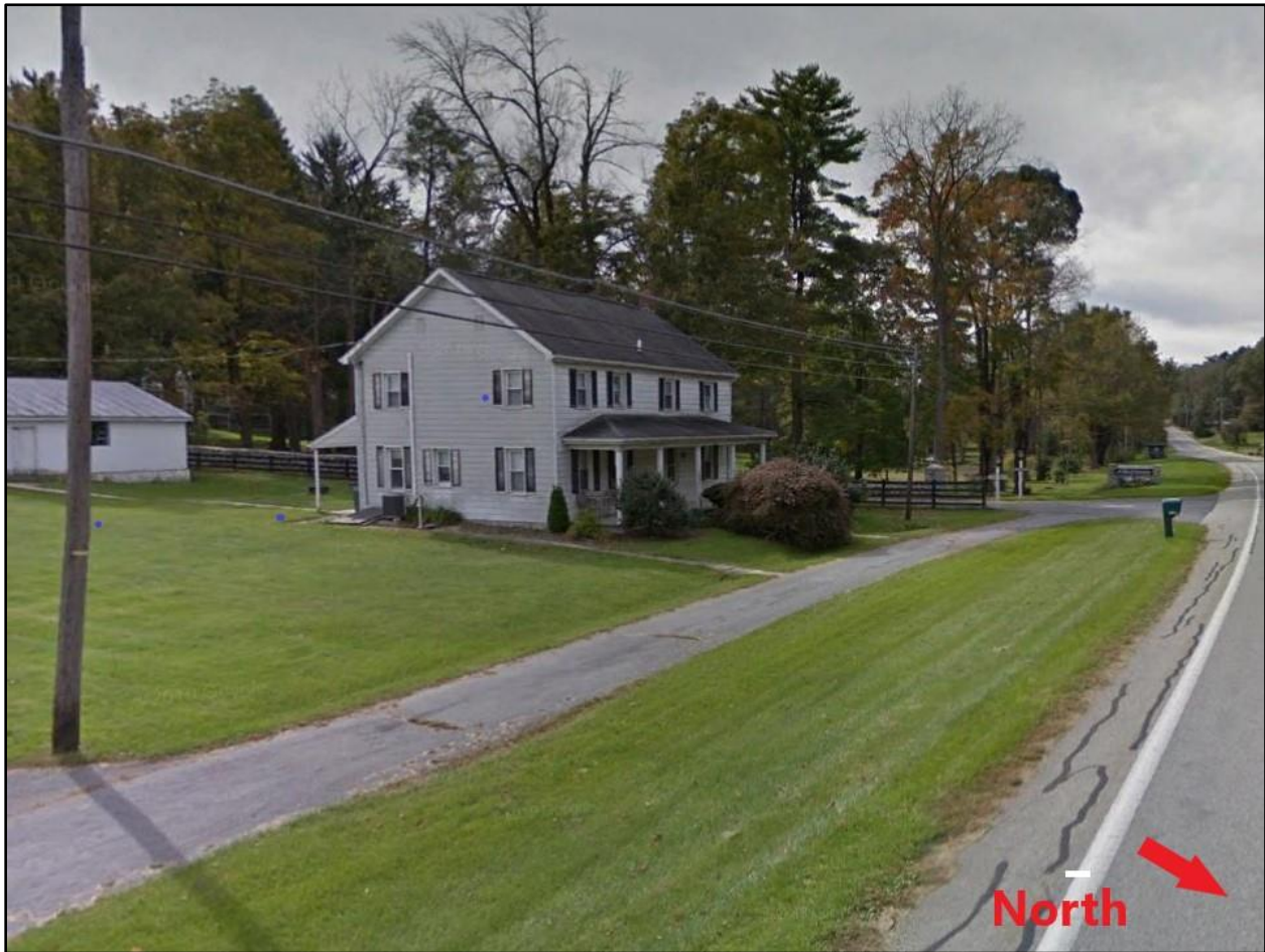
Photo 2. Sides Alpha and Side Bravo of the house. The service line on Side Bravo burned through during the fire. (Photo from Google Maps)
