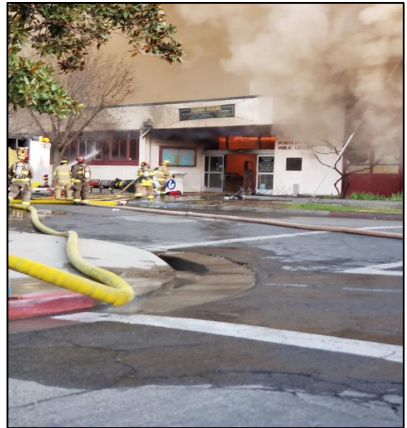
Fire Structure Side Alpha (Photo Courtesy of City Building Inspector)
