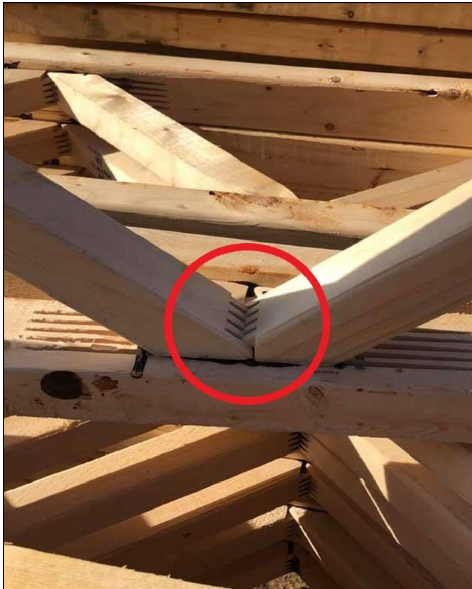
Photo 2. An example of finger joints that are precut into the chords and web members (Photo courtesy https://www.fireengineering.com/fire-prevention-protection/firefighters-and-construction-finger-jointed-wood-truss/ by Salvatore Ancona)
