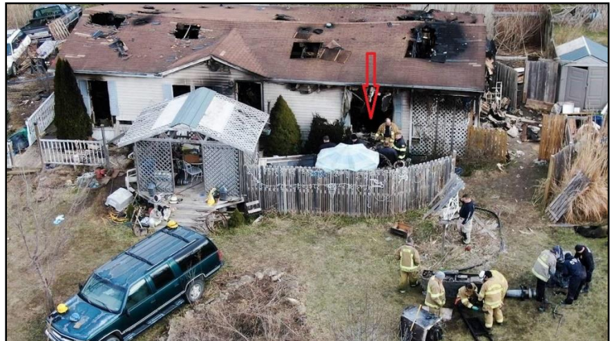
The deceased firefighter was operating a hoseline in the kitchen when the kitchen floor collapsed into the basement. The red arrow indicates the kitchen area. (Photo courtesy of the fire department.)
