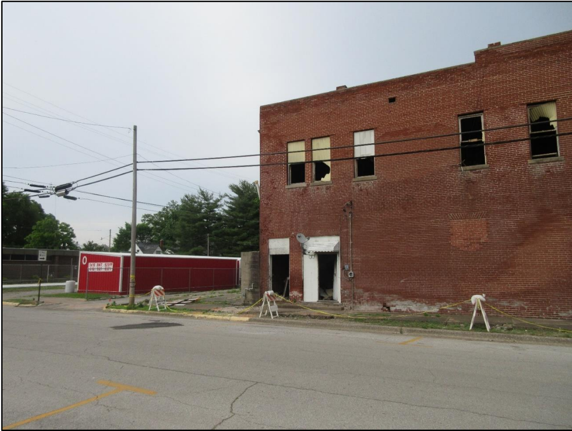
Photo 5. Side Bravo north and south doors, shown left to right. Engine 201 firefighters placed a ground ladder to the completely cleared window on the 2 nd floor.
