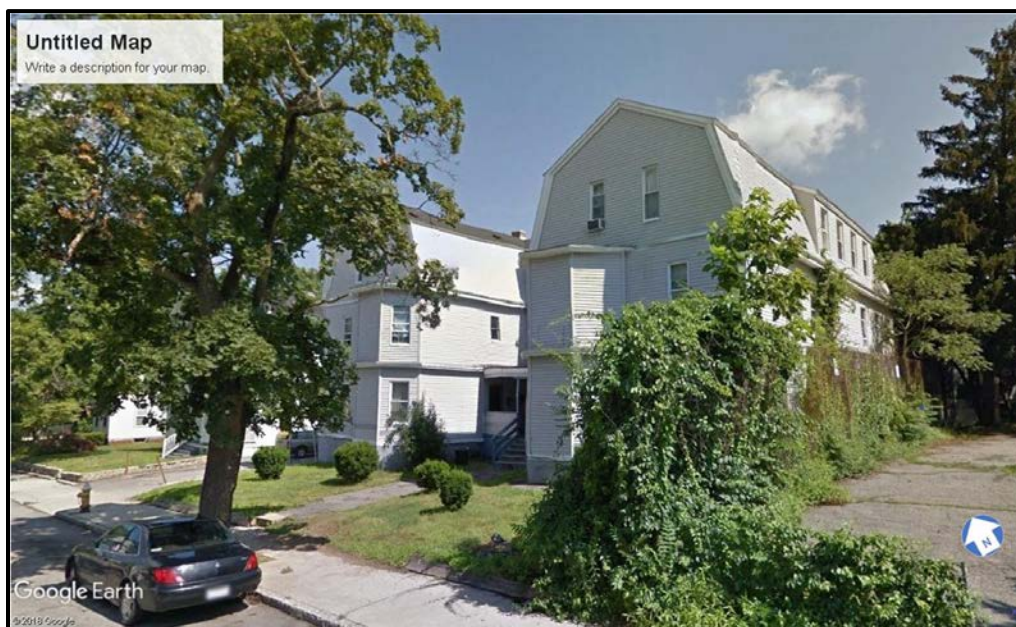
Photo 3: Side Alpha/Side Delta of the apartment building. The fence on Side Delta connected to a fence along Side Charlie. The only access to the rear of the building was from Side Bravo. (Photo adapted from Google Earth.)
