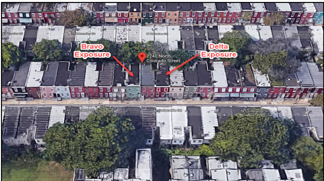
Appendix Photo 1. Street Photo: Analysis Diagram Courtesy of Buildingsonfire.com | C.J. Naum Map Courtesy of Bing Maps | Photo Courtesy of Google Earth
