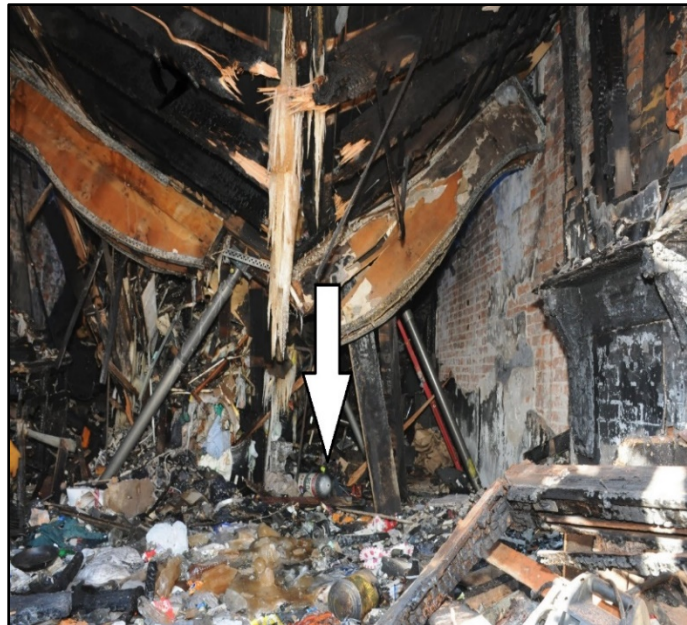
The Lieutenant was killed in a V-shape collapse while fighting a row house fire. Arrow points to victim's SCBA and the approximate area where the victim was trapped.
