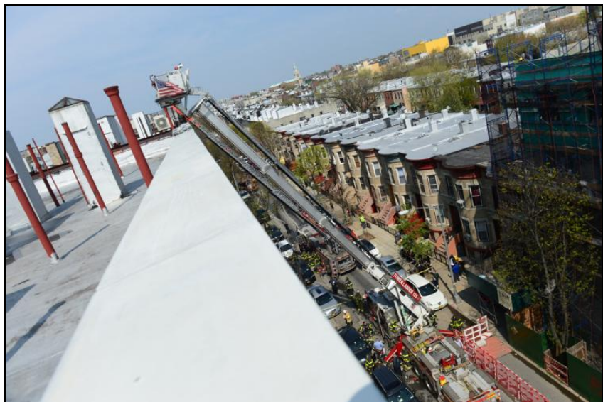
Tower Ladder 135 above the inside portion of the parapet wall. The platform jerked upwards after being released from the parapet wall ejecting the TL135 fire fighter from the platform.
