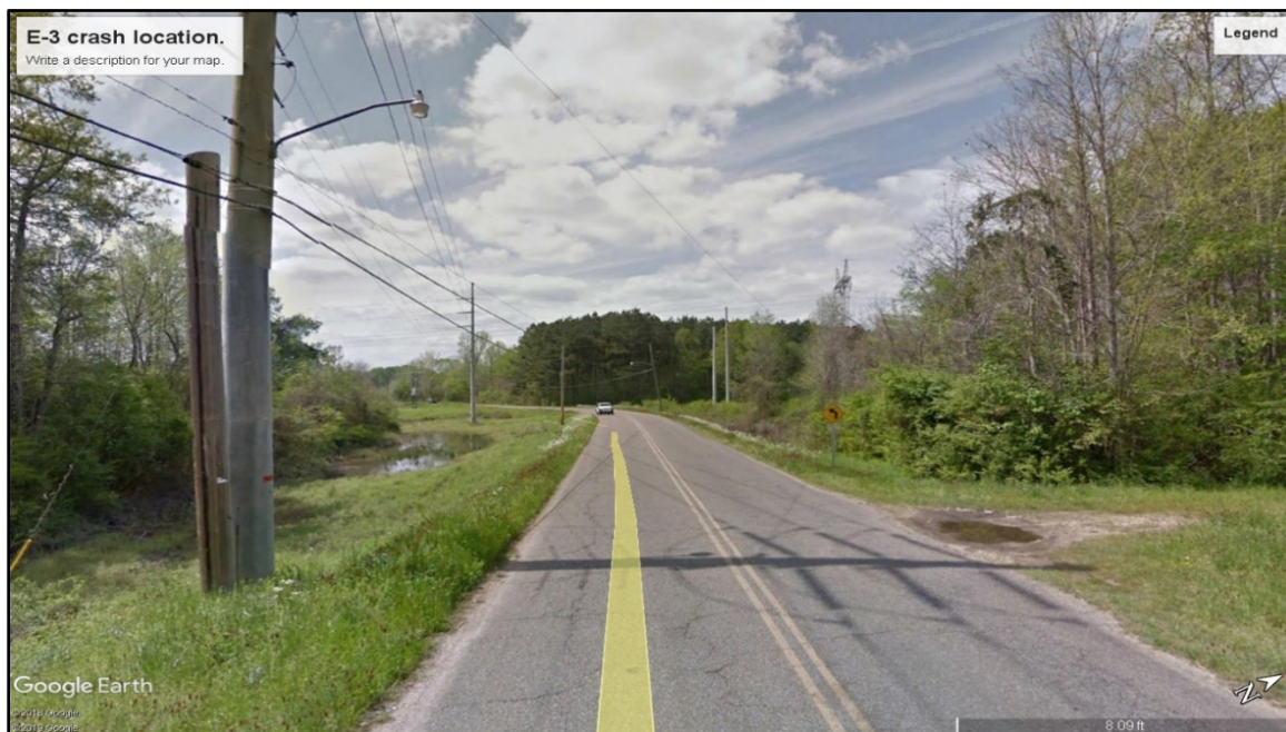
Photo 7. Curve ahead sign, but no recommended reduction in speed limit for the curve, courtesy Google Earth.
