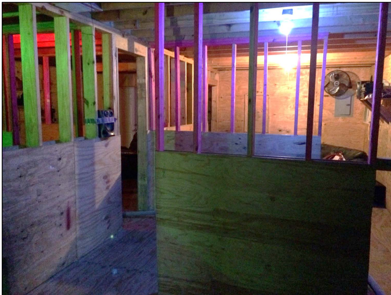
Photo 5. SCBA skill house (instructors can monitor progress by openings in interior walls). (NIOSH photo.)
