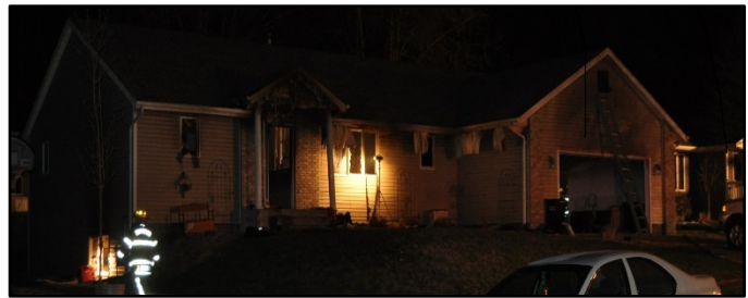
Fire structure. (Courtesy of Fire Marshall.)
