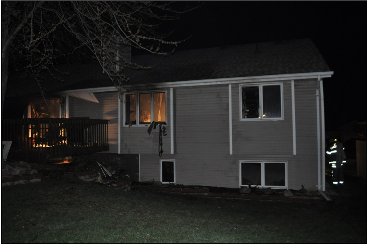
Photo 2. Partial Side C view of fire structure. (Courtesy of the Fire Marshall's Office.)
