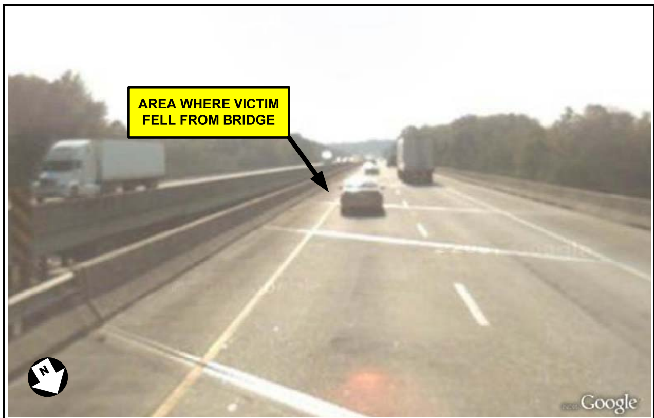
Photo 1. View travelling westbound on the highway bridge where incident occurred. Depiction from Google Earth
