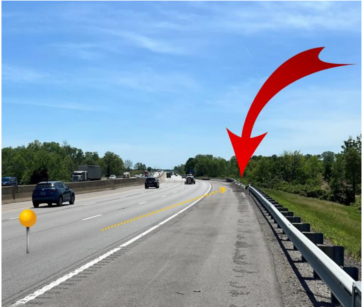
Photo 5. Photo showing victim's lane of travel (yellow location marker), direction of travel after initial strike (yellow dotted arrow), and final rest/damage to guardrail (red arrow). Photo property of Kentucky FACE.
