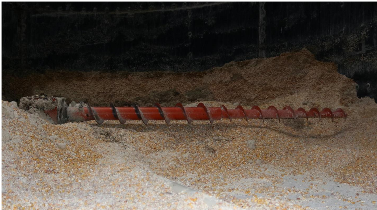
Photo 3. The unguarded sweep auger was mounted in the gearbox 8 inches above the silo floor (Courtesy of NYCAMH/NEC).
