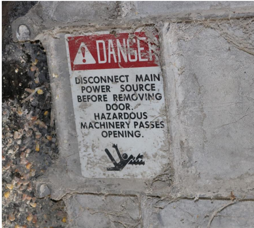
Photo 5. The warning sign on the silo hatch door requires that all operators disconnect the main power source before working near the unloader (Courtesy of NYCAMH/NEC).
