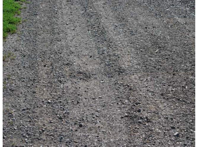
Close-up of gravel covering the orchard road.
