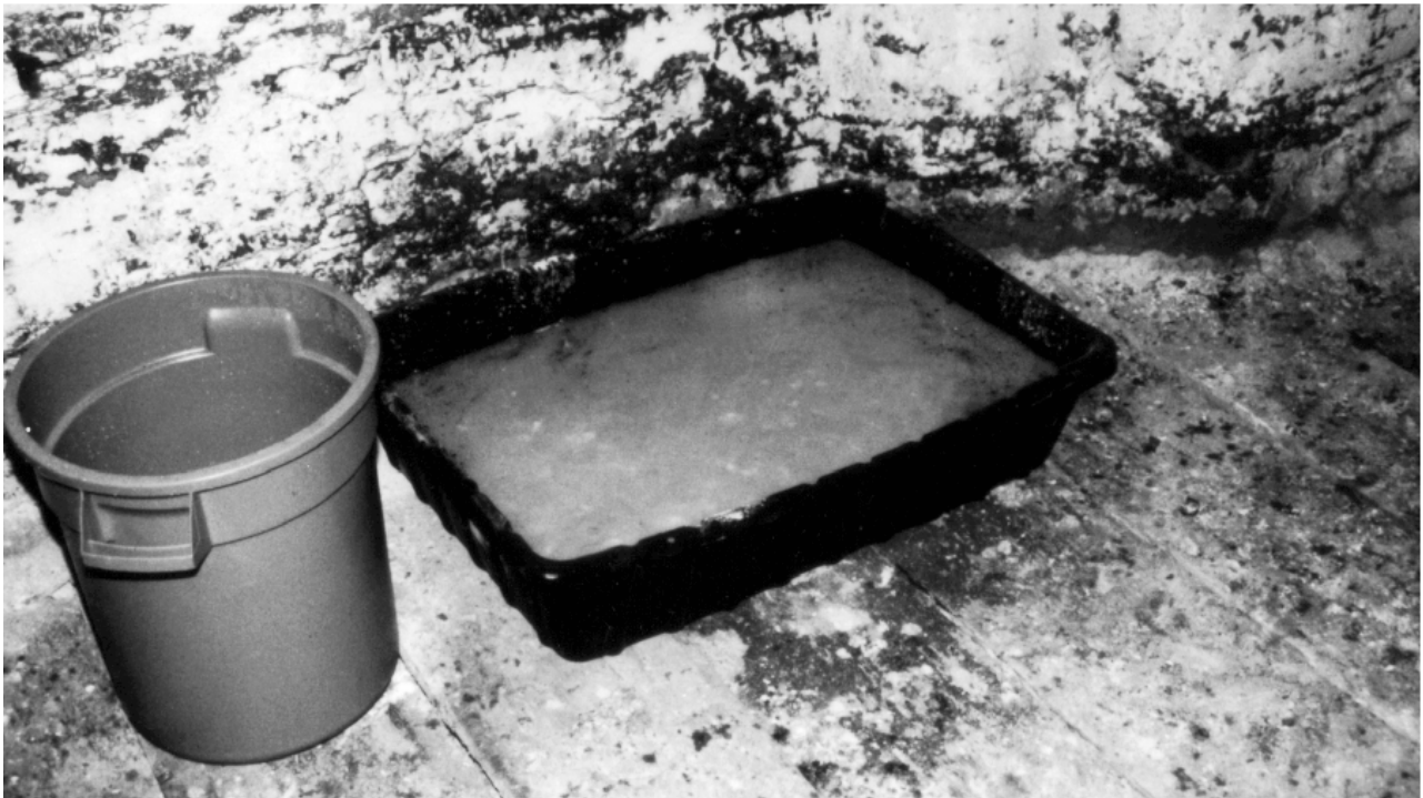
Figure 6.—Gel in tub in underground mine.
