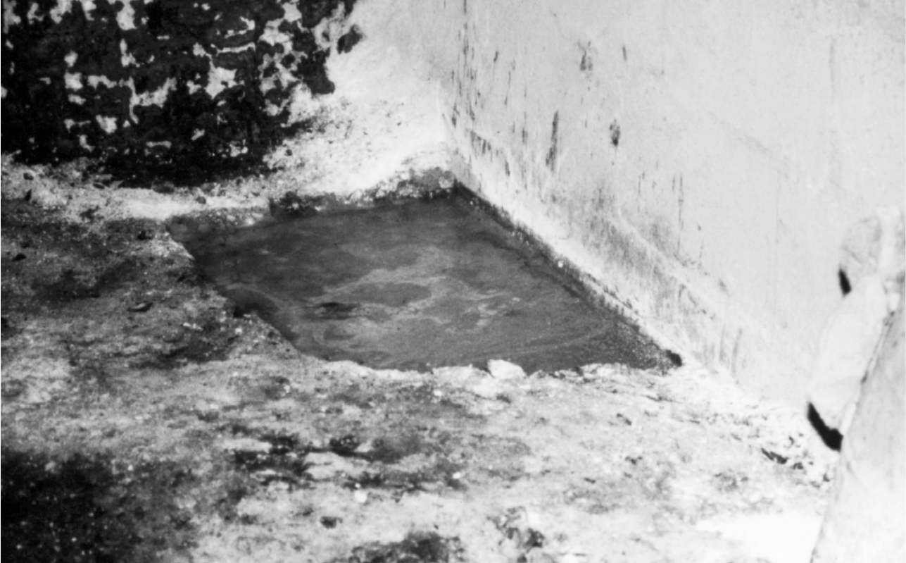
Figure 8.—Appearance of the gel after 3 months in pit in mine floor.
