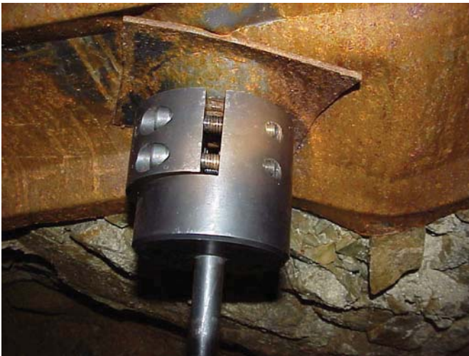
Figure 2.—Installation of pull claw on friction bolt.
