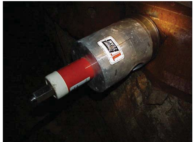
Figure 3.—Complete test assembly installed on friction bolt.
