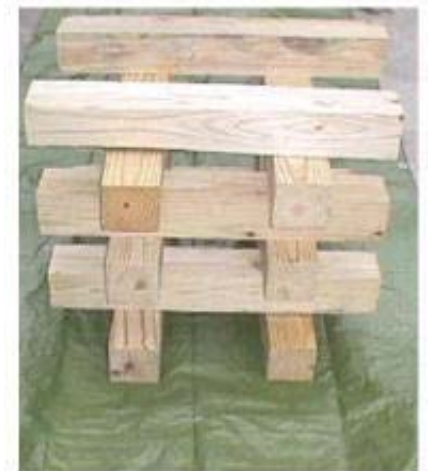
Figure 2. Example of cribbing
