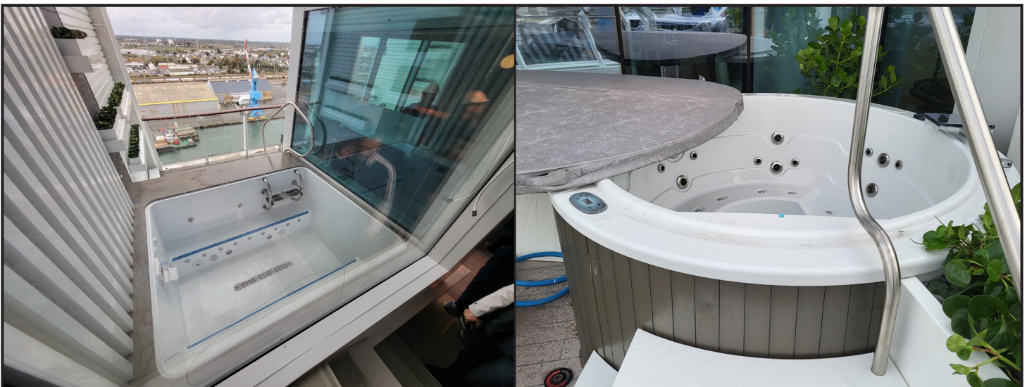
FIGURE 2. Images of hot tubs associated with cases of Legionnaires disease located on balconies only accessible via private cruise ship cabins* — two cruise ships, November 2022–July 2024
