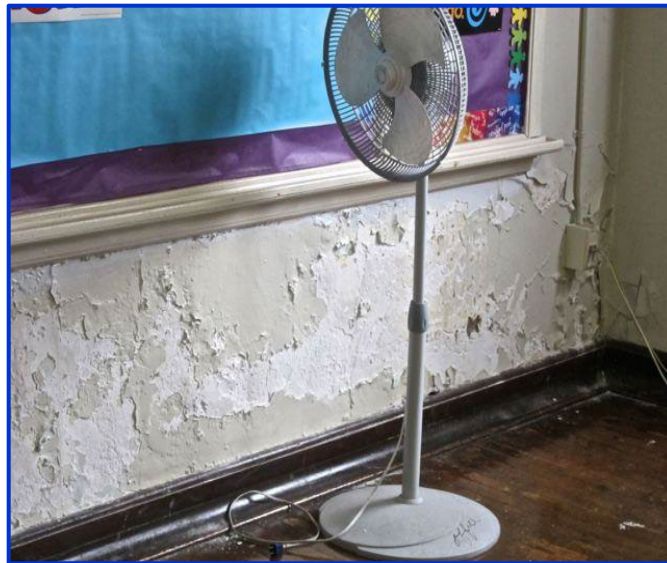
Flaking lead paint from pipes and walls
