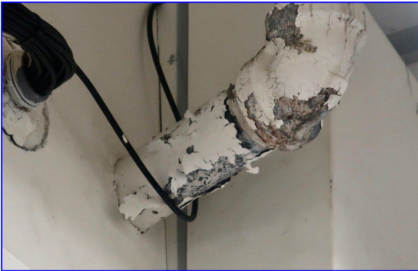
Flaking lead paint from pipes and walls
