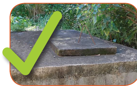
Septic tank with concrete cover
