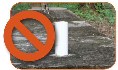
Cover ventilation pipes
