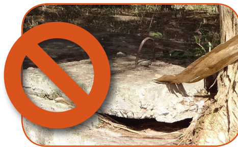
Repair broken septic tank covers
