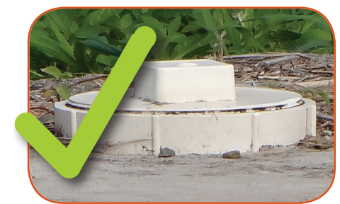
Septic tank sealed with PVC cap
