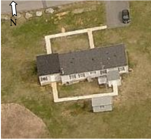
Figure 2(a). Aerial view of the house.
