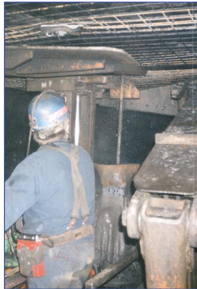
Roof screen provides overhead protection to the bolter operator during the entire bolting installation process.
