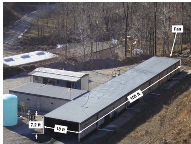
Figure 1. Fire Suppression Facility.
