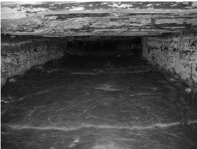
Figure 13. Photo taken 8-16-07 looking inby at study site, location 1.
