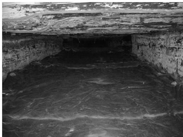
Figure 4. Photo of roof rock collection areas 8-16-07, location 1.
