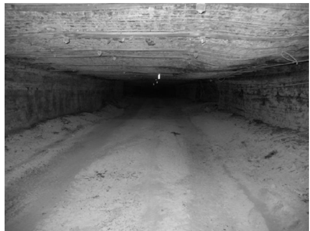
Figure 15. Photo taken 6-25-08 looking inby in adjacent entry with screen, location 15.
