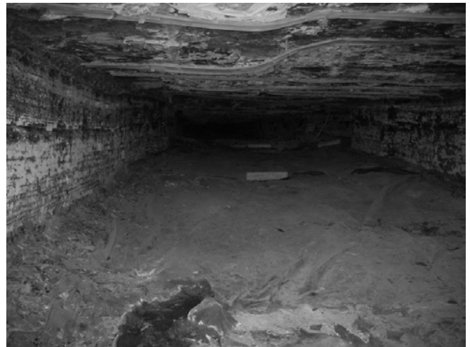
Figure 14. Photo taken 6-25-08 looking inby at study site, location 1.
