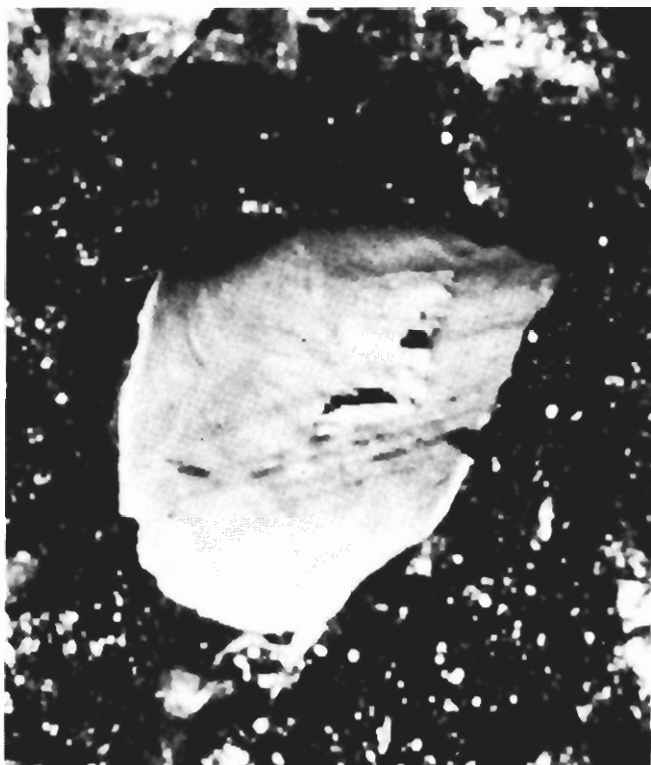
FIGURE 9. - Hole 2 after mine-through, April 10, 1980, showing calcite lining the lower half of the hole. Location A (fig. 8).
