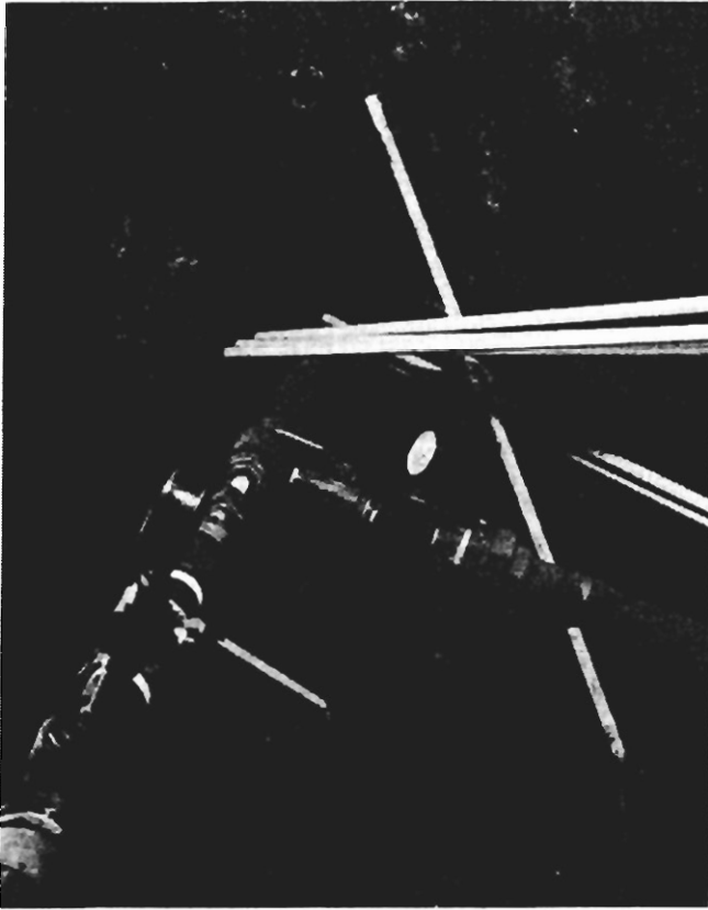
FIGURE 7. - Second view of hole 2 during flushing operation. Note 12.7-mm (0.5-in) PVC pipe in background.
