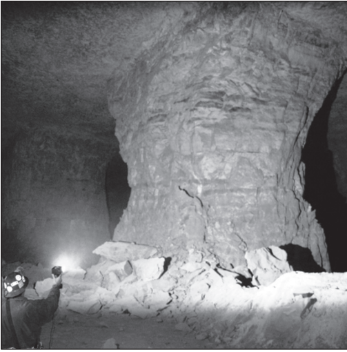
Figure 3. Partially benched pillar failing under elevated stresses at the edge of bench mining. Typical hourglass formation indicating over-loaded pillar.
