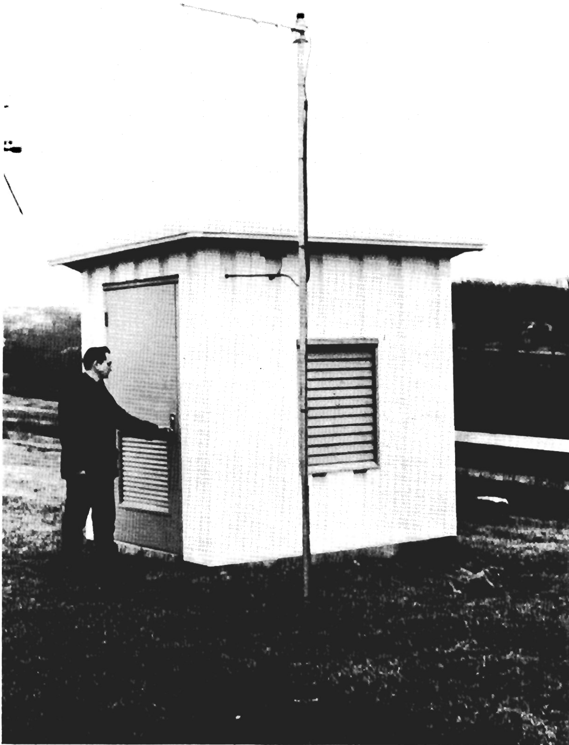
FIGURE 20. - Surface transmitter-receiver-antenna station for overland radio loopback.
