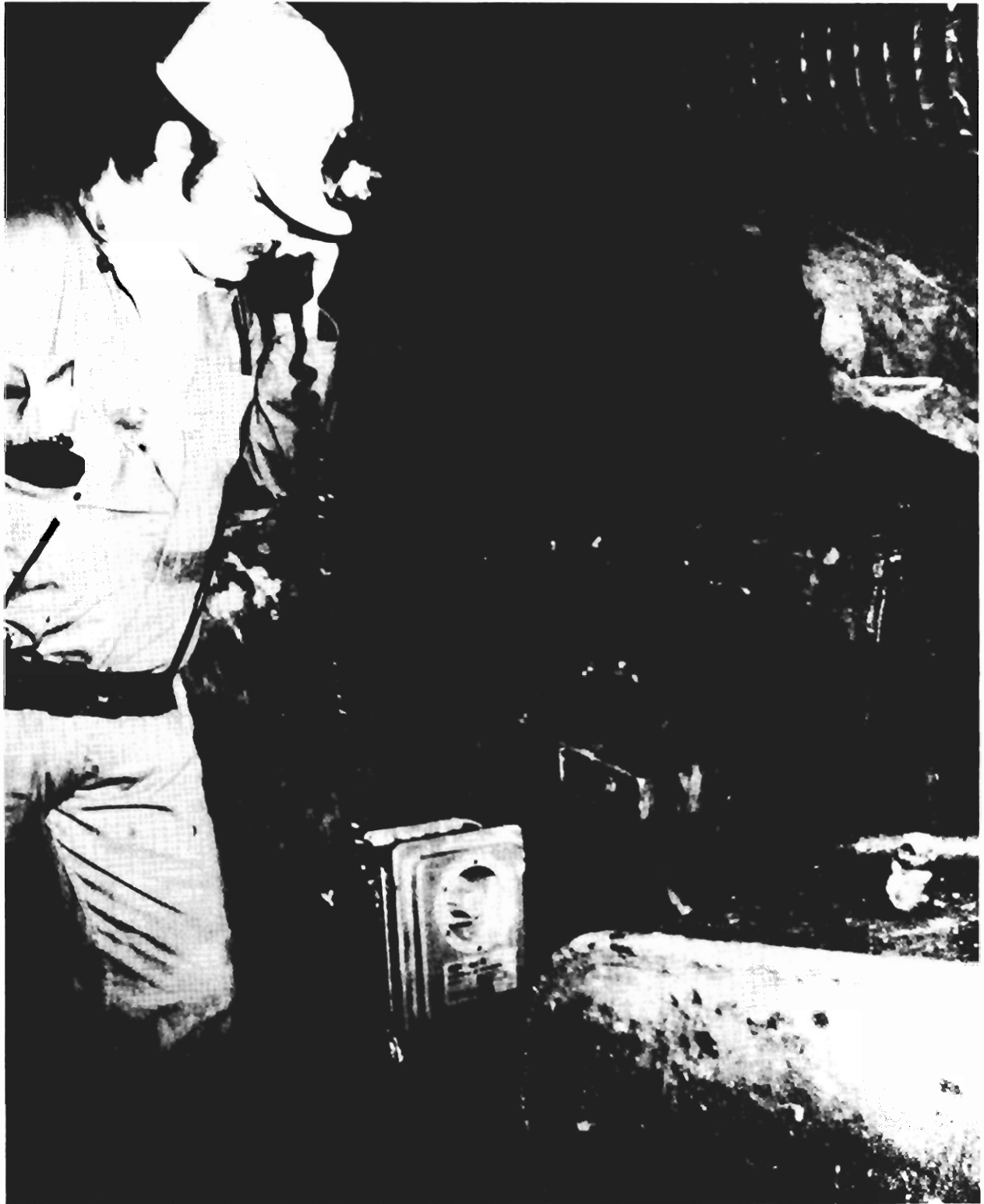
FIGURE 2. - Loudspeaking phone on roof bolter.
