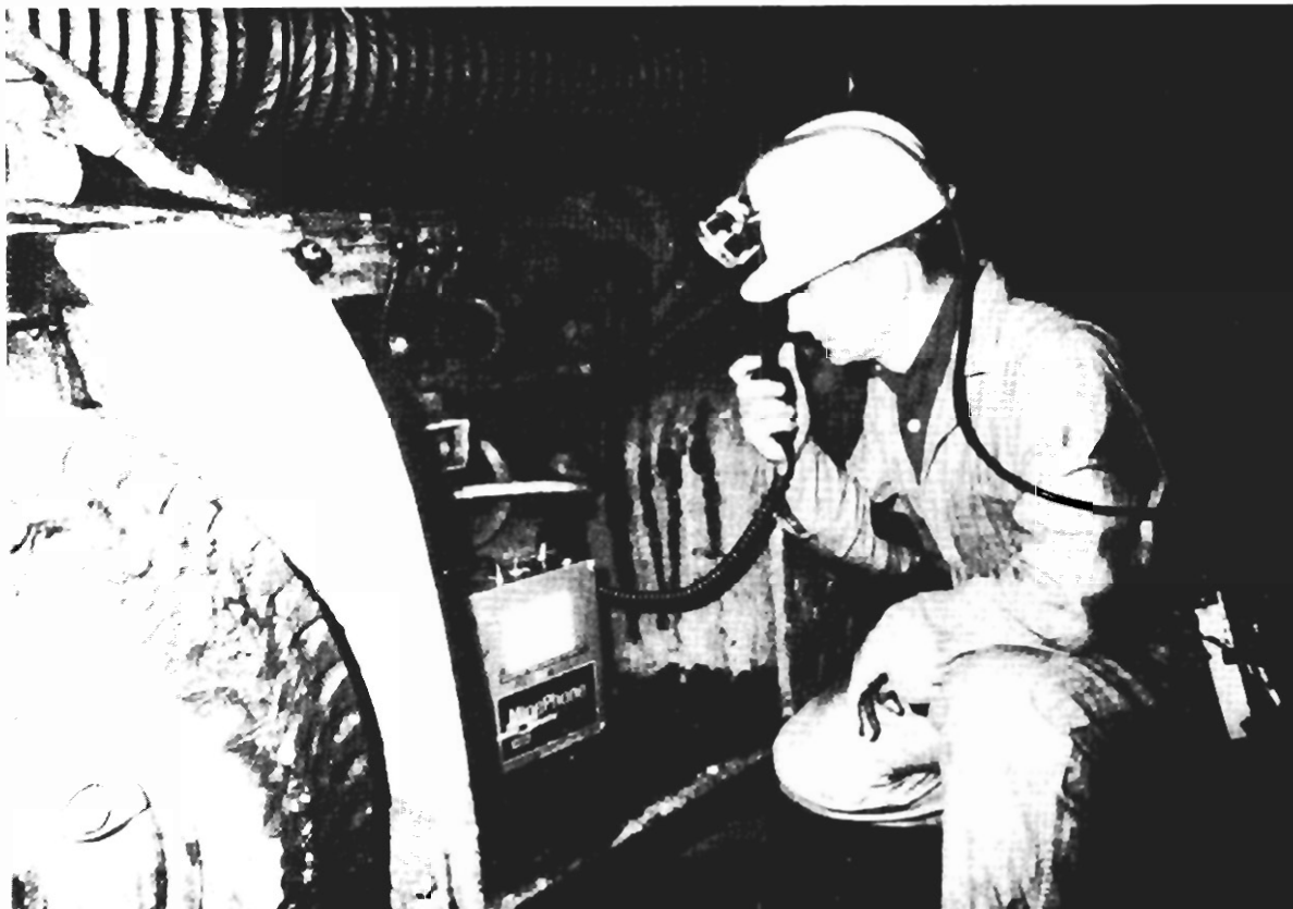
FIGURE 7. - Carrier phone on face machine.
