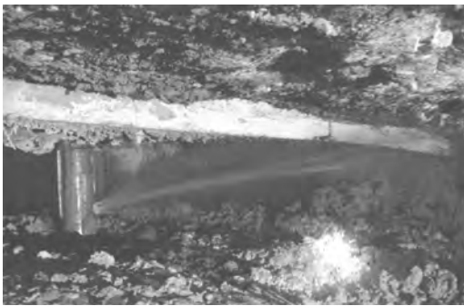
Figure 6. Use of spray nozzle during mine seal construction.
