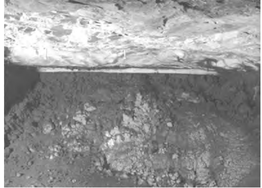
Figure 7. View of completed mine seal.
