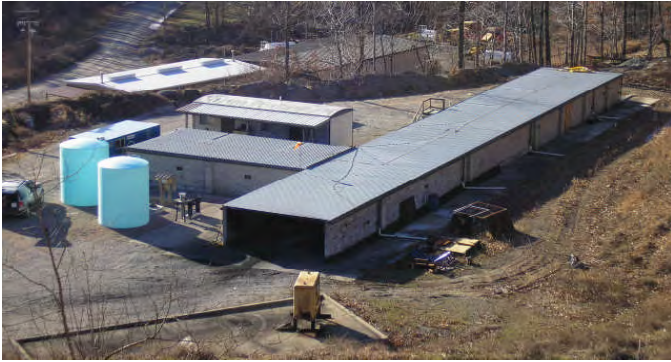
Figure 1. Fire Suppression Facility.
