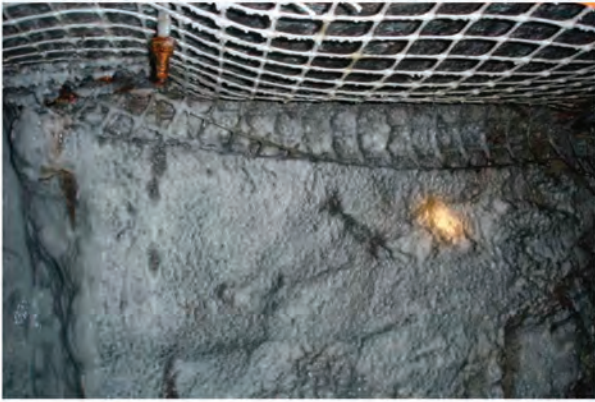
Figure 3 — Roof and rib 48 hours after gel application.
