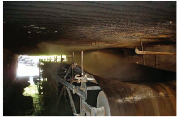
Figure 5 — Second water/Barricade II sprinkler flow test.
