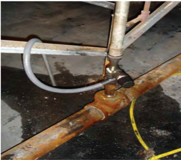
Figure 4 — Eductor in 1-1/2 in water line.
