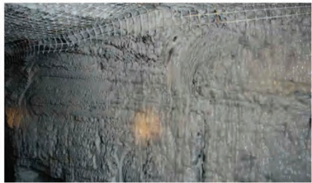
Figure 2 — Roof and rib after gel application.
