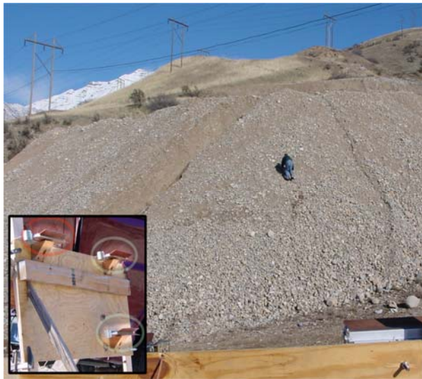
Figure 4. Radar view of slope with man climbing; inset shows transmit antenna (left) and receive antennas (right).
