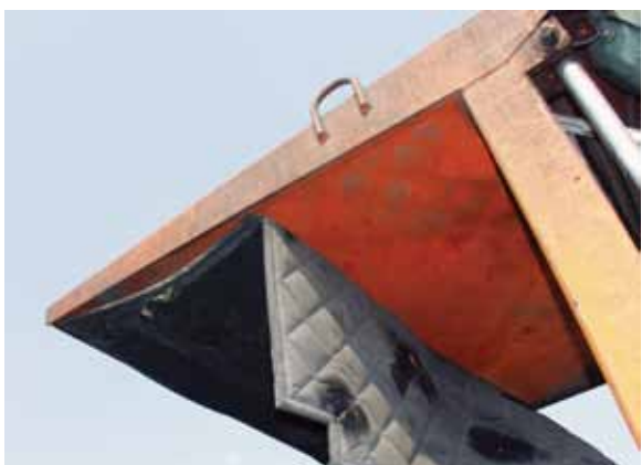
Figure 26. One-inch-thick quilted fiberglass blanket being removed for testing.
