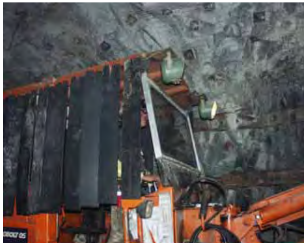
Figure 31. Windshield installed on bolter 5.
