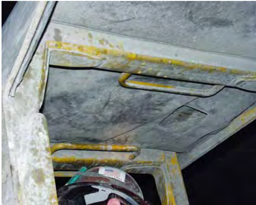
Figure 3. Haul truck with vinyl-covered material installed in canopy above the operator.
