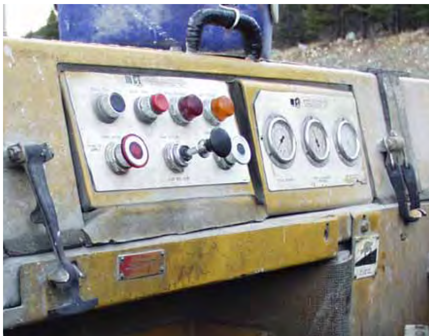
Figure 9. Gaps around instrument panel sealed with foam.
