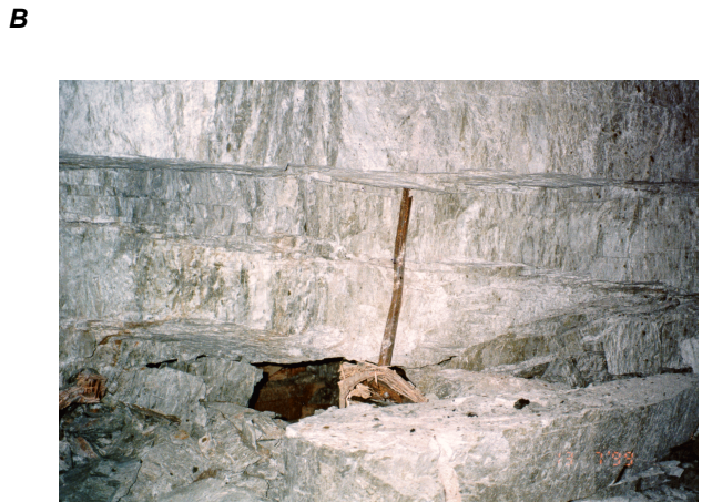
Figure 4. Cut (or drift) in a steeply dipping hard-rock vein. A, View along wall. Photo taken while standing on sandfill from previous cut. Note mining-induced fractures and temporary friction rock bolts from roof of previous cut exposed in wall. B, View of wall showing bent rock bolt offset by shear displacement along an echelon fracture zone.
