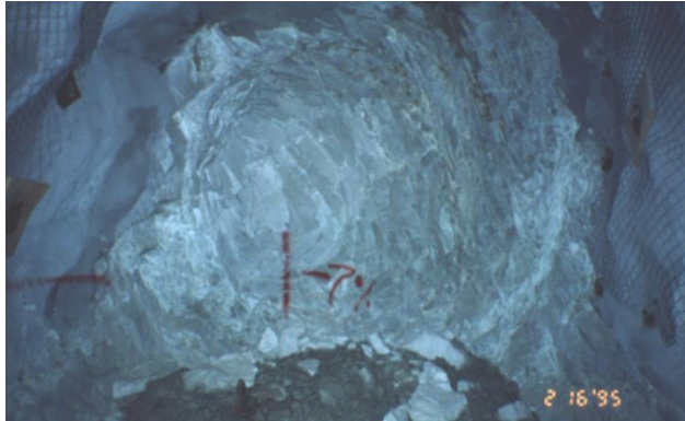
Figure 1. Cavity created by a face-strain rock burst in a development heading of a hard-rock mine.
