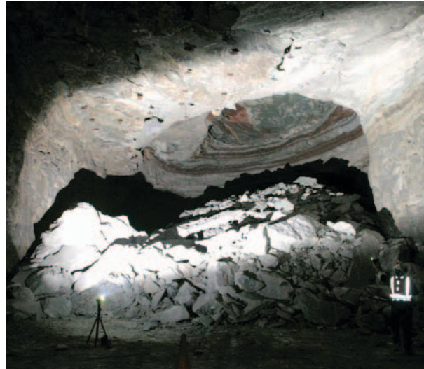
Figure 3. Example of a large elliptical-shaped roof fall that was related to high horizontal stress in the roof.
