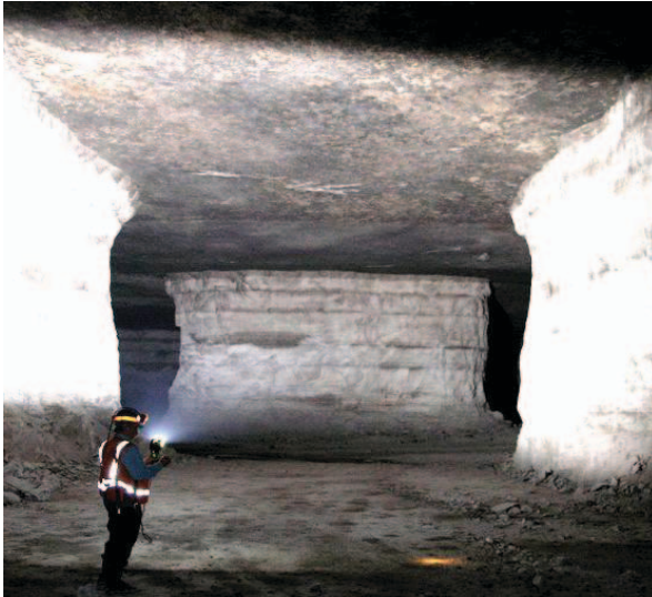
Figure 2. Naturally stable 44-ft (13-m) wide roof span in a stone mine.
