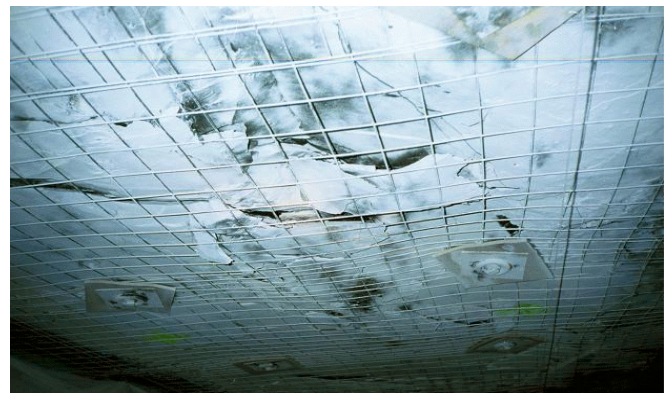
Figure 1. Roof screen effectively controlling weak roof skin.
