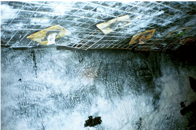
Figure 2. Roof screen achieving up to 94% roof coverage.
