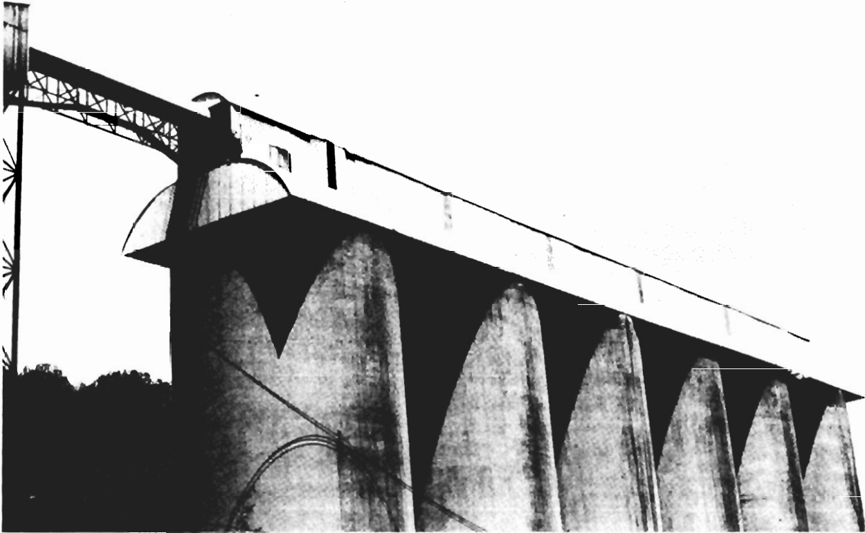
FIGURE 3. - The Nelms No. 2 cluster of open-top silos is covered by a metal roof that allows free movement of air.
