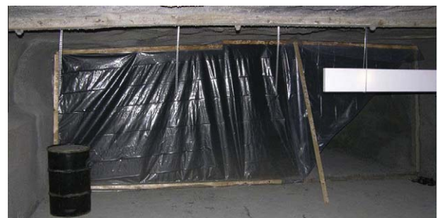
Fig. 4. Plastic diaphragm used to contain methane within the ignition chamber.
