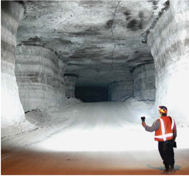
Fig. 6. Stable pillars in a limestone mine at a depth of cover of 275 m. Slightly concave pillar ribs formed as a result of minor spalling of the hard, brittle rock.
