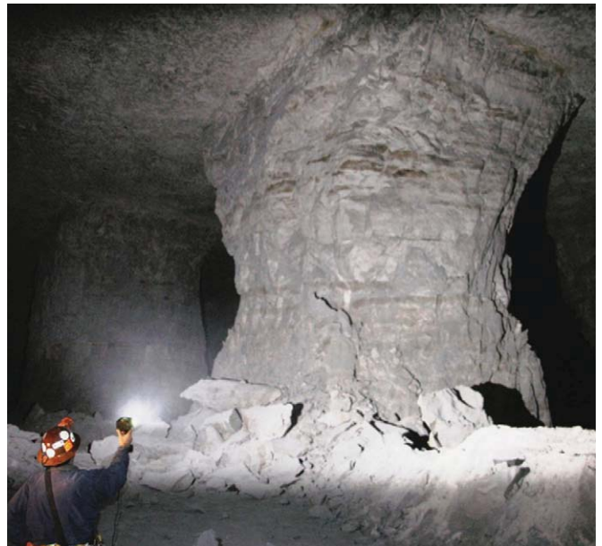
Fig. 5. Partially benched pillar failing under elevated stress at the edge of bench mining. Typical hourglass formation indicating overloaded pillar.
