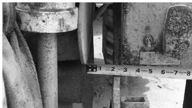
Figure 13 — Available clearance between control panel and drill platform. The clearance is approximately 63.5 mm (2.5 in.).
