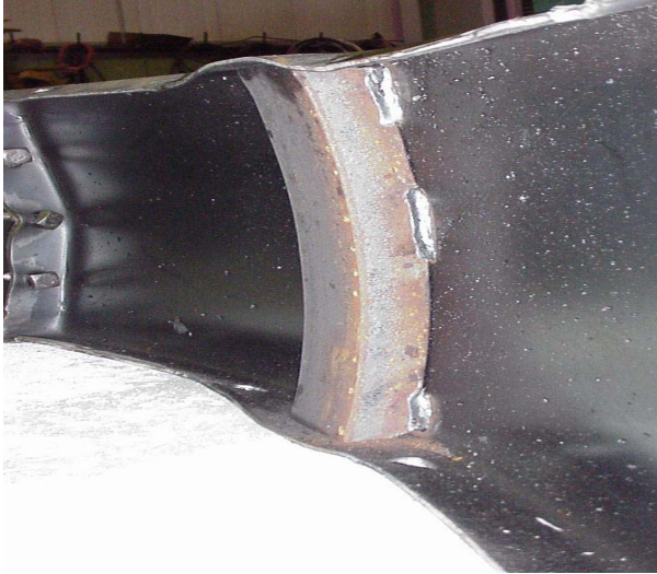
Figure 15. Buckling of steel channel in single ring test.
