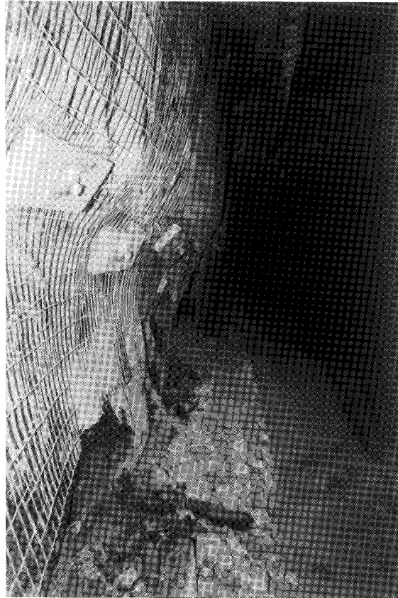
Figure 10.—Using wire mesh for rib control.
