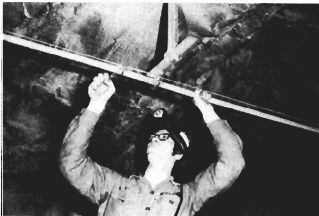
FIGURE 3-29. - Radiac cable installation on messenger wire.
